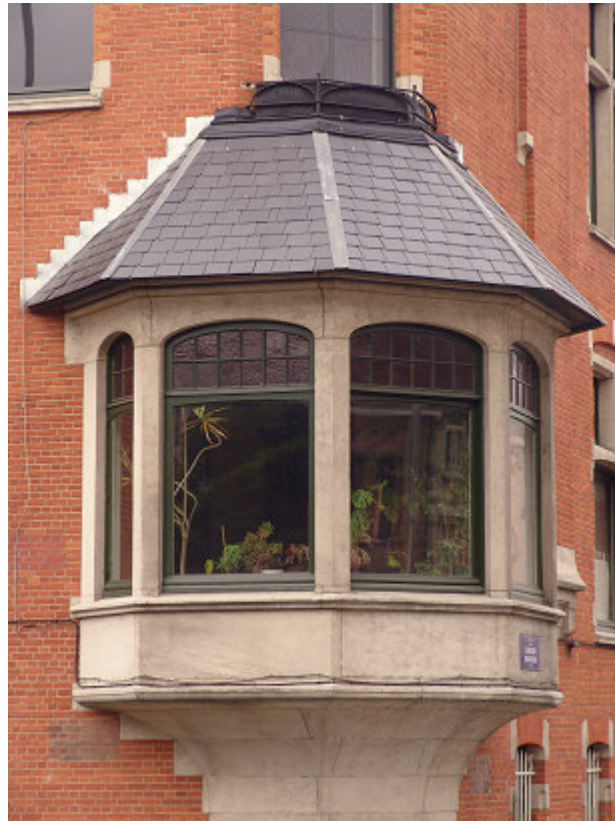
Quaker House in Brussels - The bow window on the main façade (Picture : M. Berthold)
